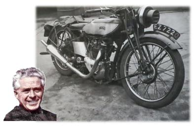
The world's first Triton, built by Rex McCandless during WW2 A racing Triumph Tiger 100 motor in a Norton International racing chassis. Note headlamp mask – required during wartime blackouts.
